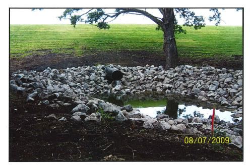
A distilling basin was constructed below the outlet structure of Thomas Mitchell Pond. This basin was designed to catch sediment from the dredging process and provide an additional sediment storage before water enters Camp Creek.
