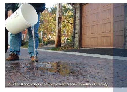
and preventing them from reaching the storm sewers. Even the stormwater that makes it into the storm sewer is cleaner than it would be otherwise," says city engineer Jon Dienst.
