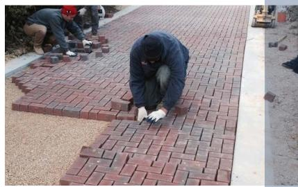
Workers install a permeable paver system in Clinton.
