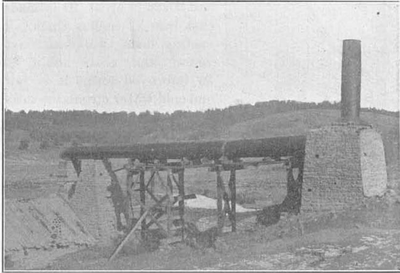
Fig. 97. Waters' lead furnace at Dubuque showing fume saving arrangement.
