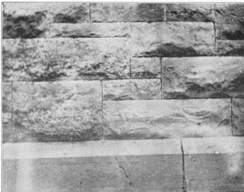
FIG. 100. Use of Galena dolomite in massive construction.
