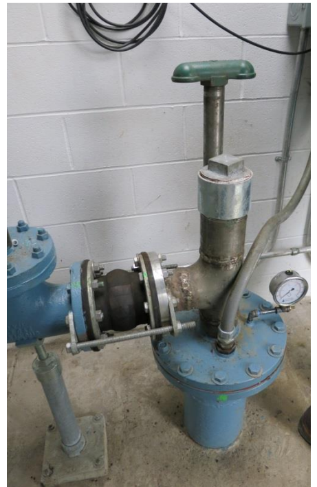
New well with vent
