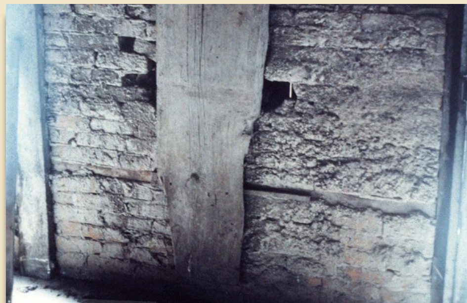
Detail of "fachwerk" construction at the Bonaparte Pottery, 13VB200.
