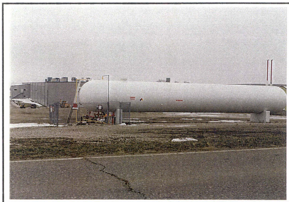
Photograph Description View to the south of 30,000-gallon LP AST Figure No. 4-1 (owned and operated by Star Energy LLC) at SMITHCO, 11-30-00.
