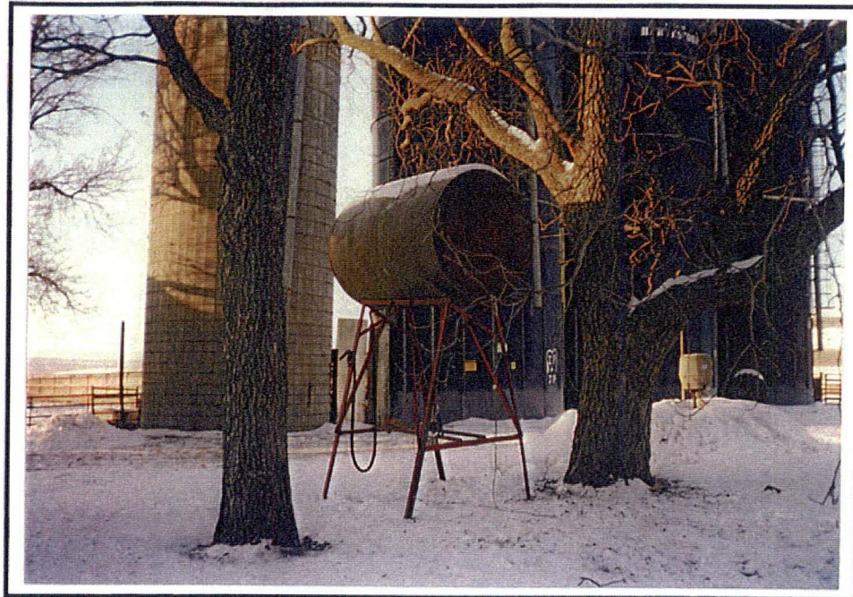
Photograph Description View to the south of (1)500-gallon gasoline AST Figure No. 4-1 at the Probst Farmstead, 1-3-01.
