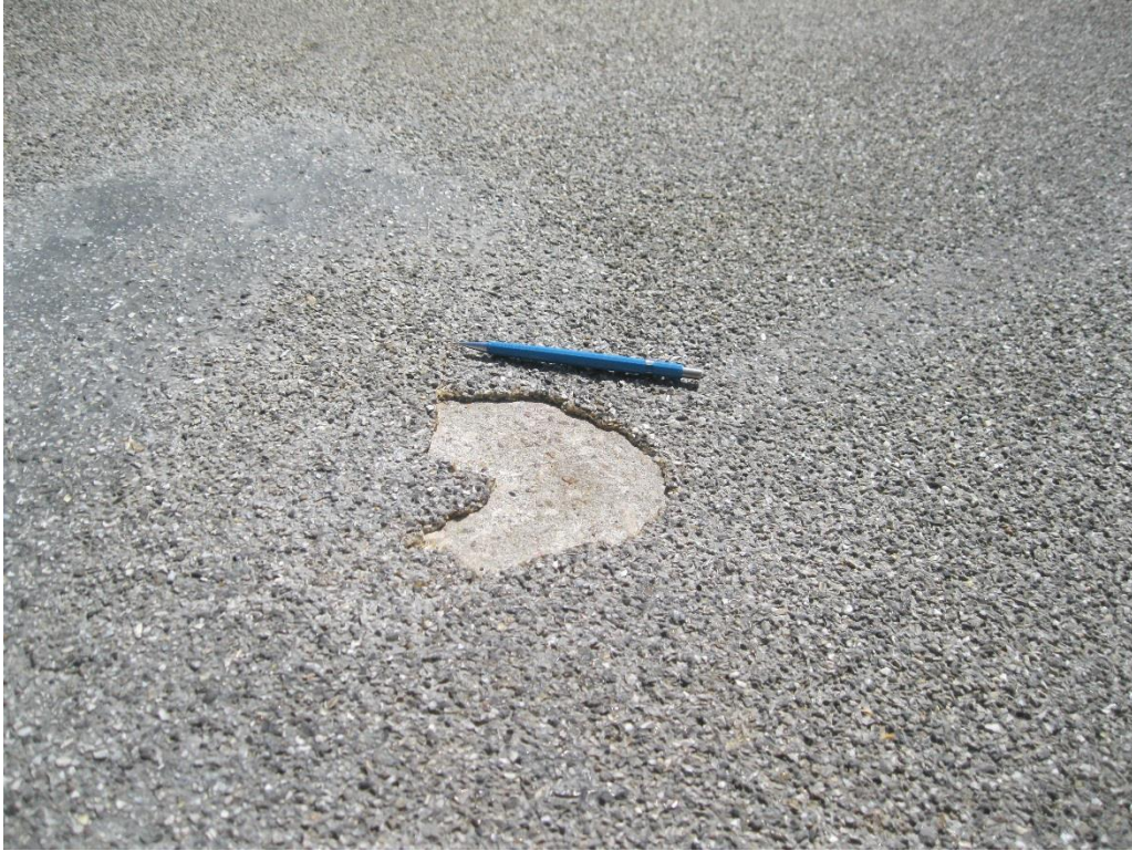
Figure 61. Johnson County close-up of exposed concrete deck in southbound lane
