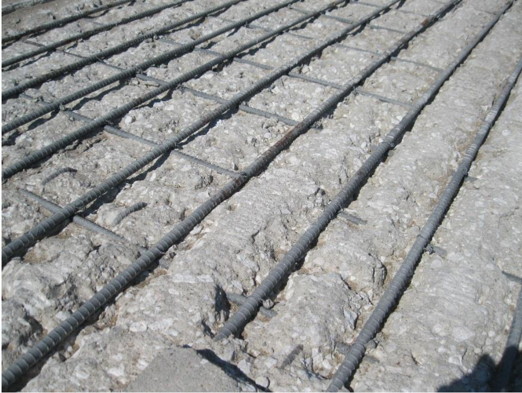
Figure 18. Exposed reinforcing steel bar condition on Johnson County bridge
