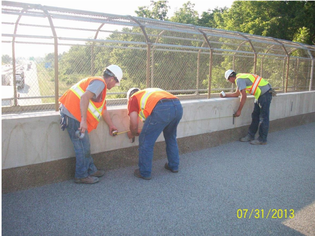
Figure 33. Marking Johnson County barrier rail
