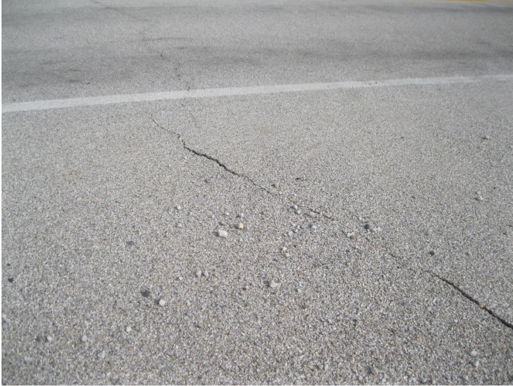
Figure 74. Keg Creek reflective cracking in approach slab
