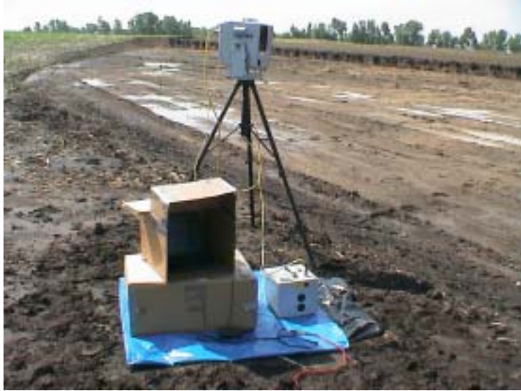
Figure 16. Equipment Protected Using a Tarp and Boxes (Borrow Pit)
