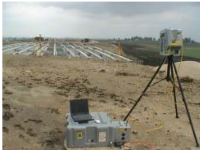
Figure 11. Hardin County Bridge Facing East (Bridge Beams)
