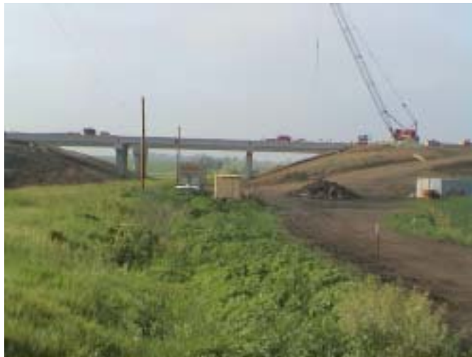
Figure 10. Hardin County Bridge Facing South (Bridge Beams)
