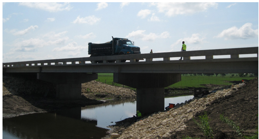
Live load testing on the completed bridge
