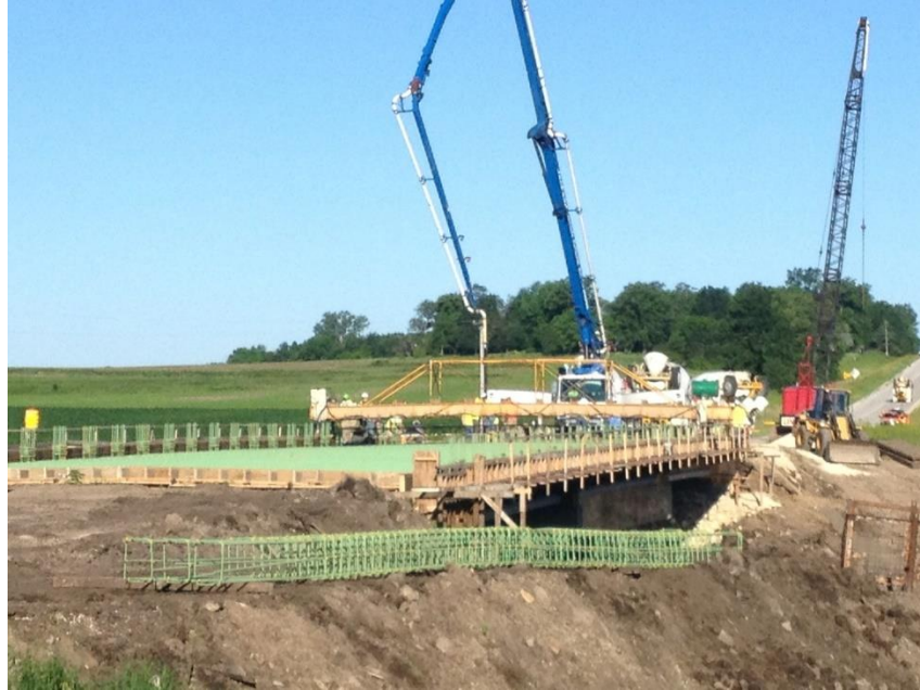
Figure 3. Three-span bridge at Pine Creek during concrete placement
