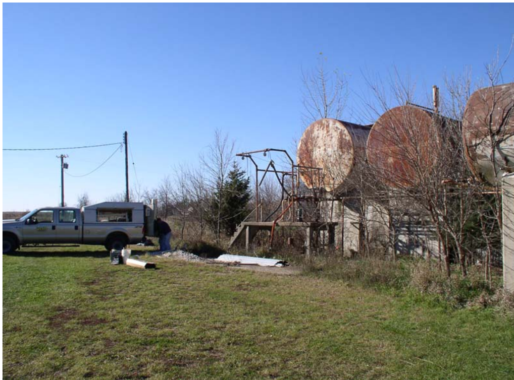
Photo 2 – View of Former AST Bulk Plant from the Northeast
