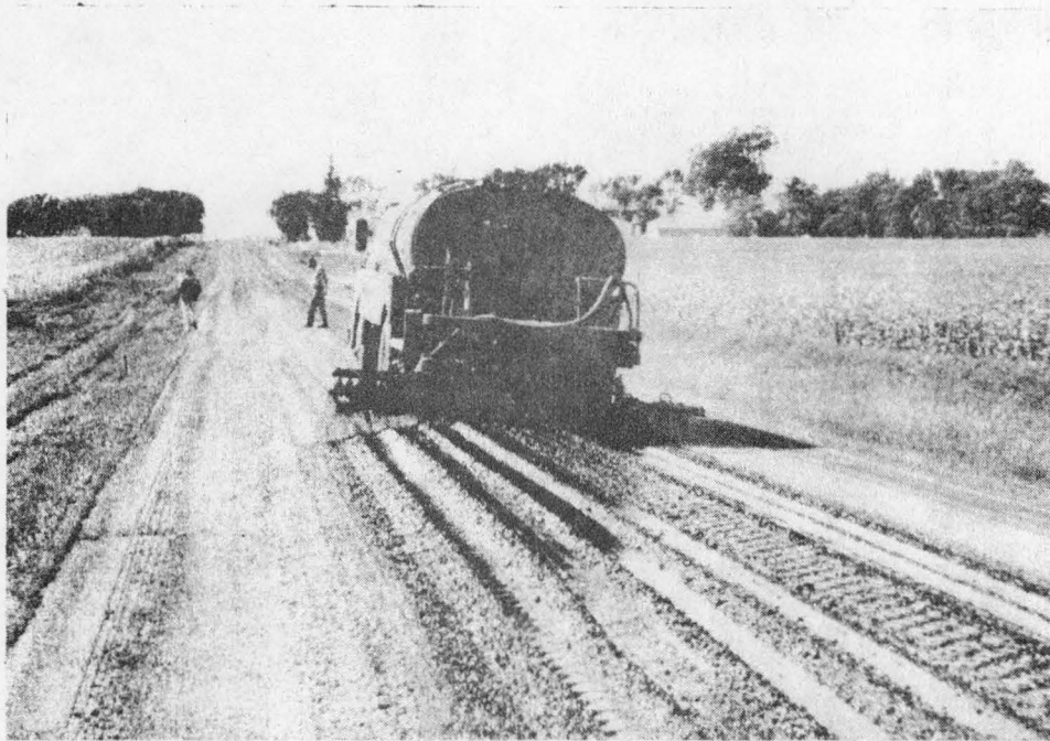
Figure 3. First application of SC-800 to road mix
