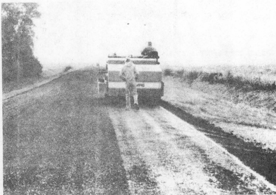
Figure 6. Compaction of road mix section
