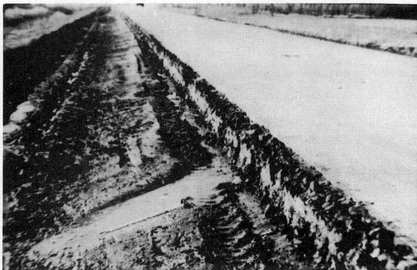
Figure 8: Drainage Through Macadam Base
