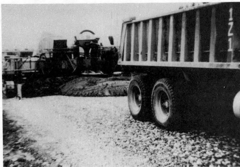
Figure 7: Concrete Truck on Macadam Base
