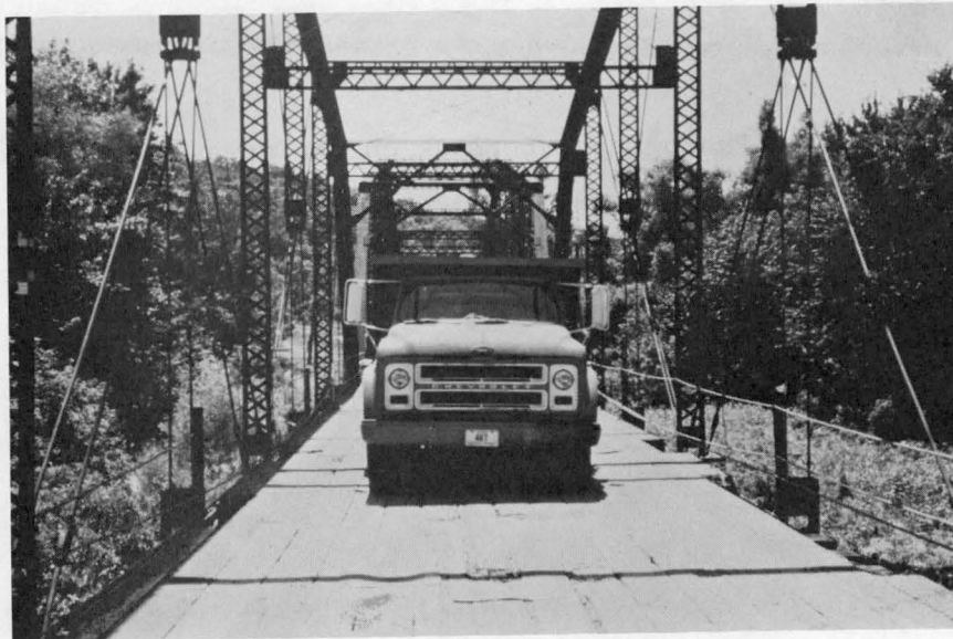
Fig. 13. Photograph of truck on the centerline of the bridge.
