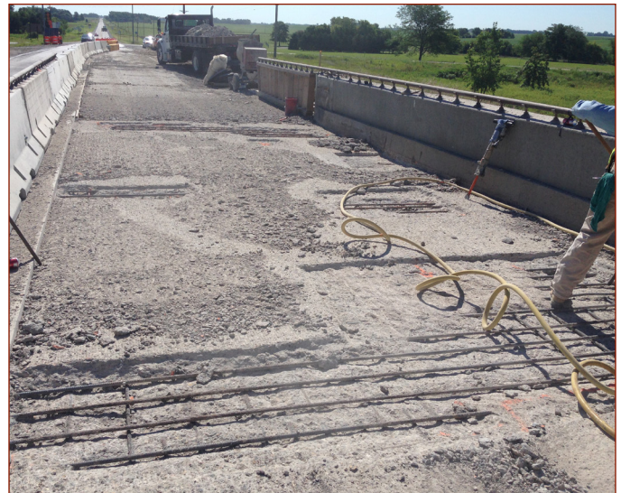
Overlay construction site showing extent of in-depth substrate concrete removal
