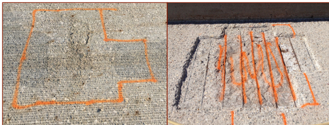
Area marked for additional substrate concrete removal after milling and cleaning top of the deck (left) and an area marked for more in-depth concrete removal (right)
