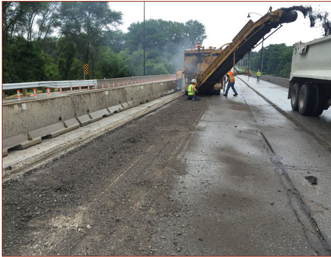
Use of milling machine to remove top layer of bridge deck
