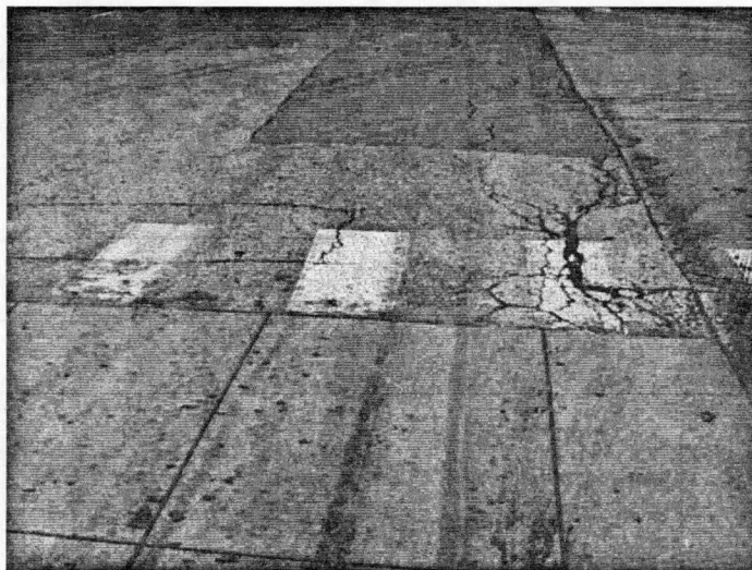
Figure 2. Deteriorated Asphaltic Concrete Surface
