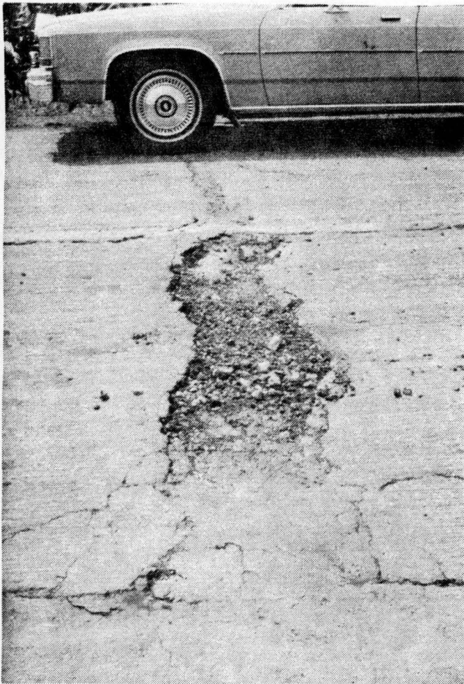
Slippage Crack Replaced
