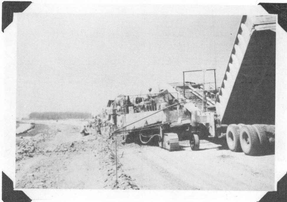
Batch truck dumping wet cement at site. PC Pave - 1985
