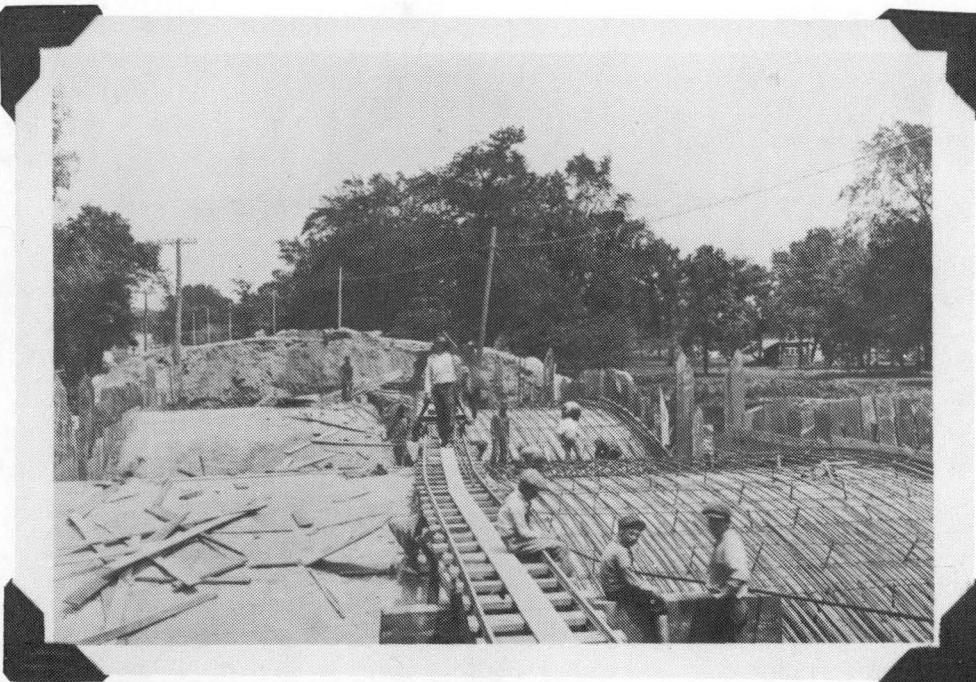
Hand tied reinforcing bar. Hand pushed board carried bars and wet concrete to floor of bridge on narrow gauge tracks. (Head)
