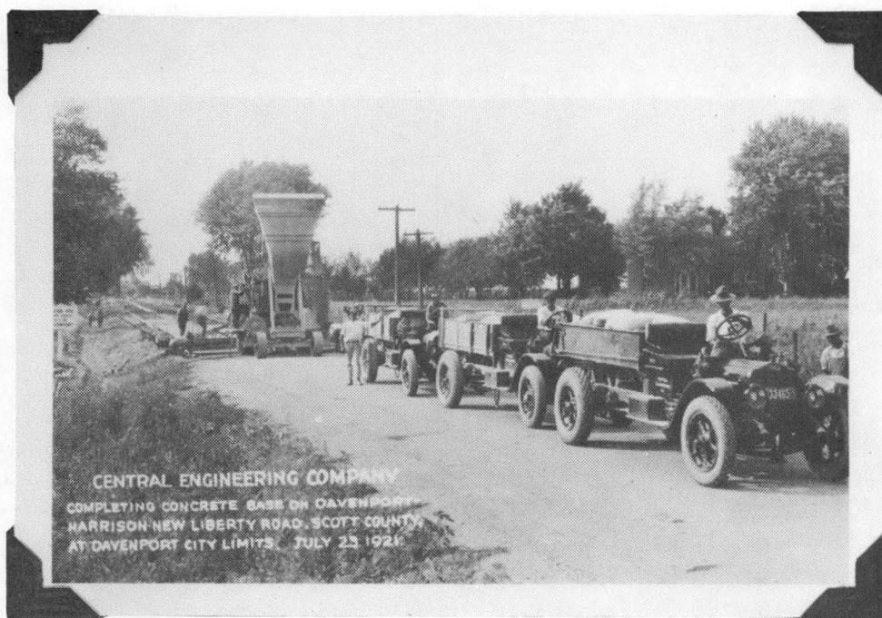
Concrete base work on New Liberty Road in Davenport - 1921
