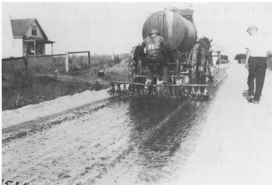
(Left) Early seal coating. (Below) Another view of highway construction at Guthrie Center.
