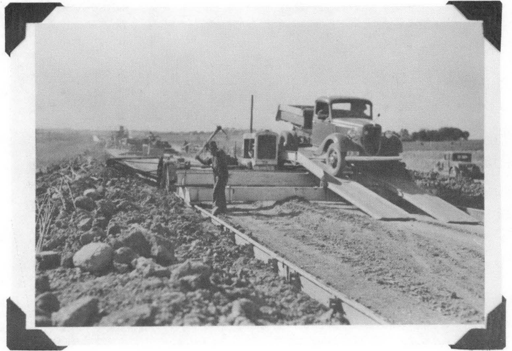
Paving 1930's - Truck backing up over subgrade shaper to go back to paver.
