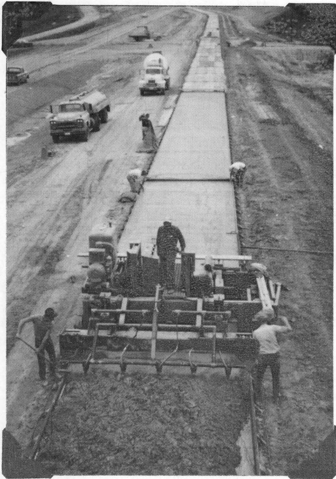
Paving 1960's - Smoothing wet concrete in front of finishing machine. Finished slab behind.
