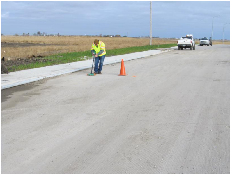
Figure 4. Testing at the South Bound Rest Area Car Parking
