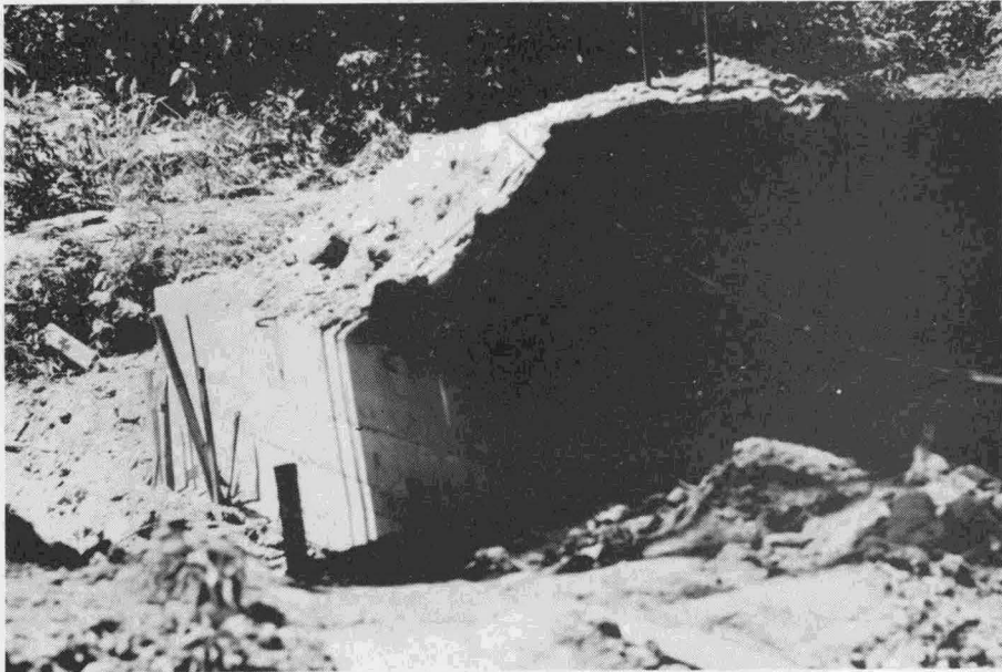
Fig. 25. Photograph of concrete mat with soil.
