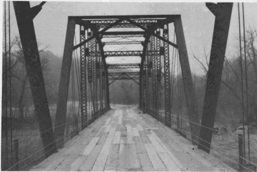
Fig. 1. Photographs of the Hubby Bridge.
