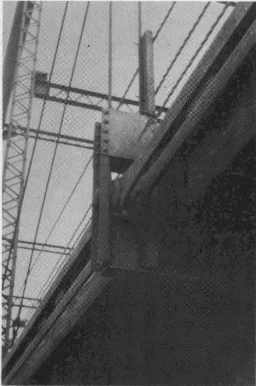
Fig. 4. Photograph of typical connection of floorbeam to truss at hanger member.
