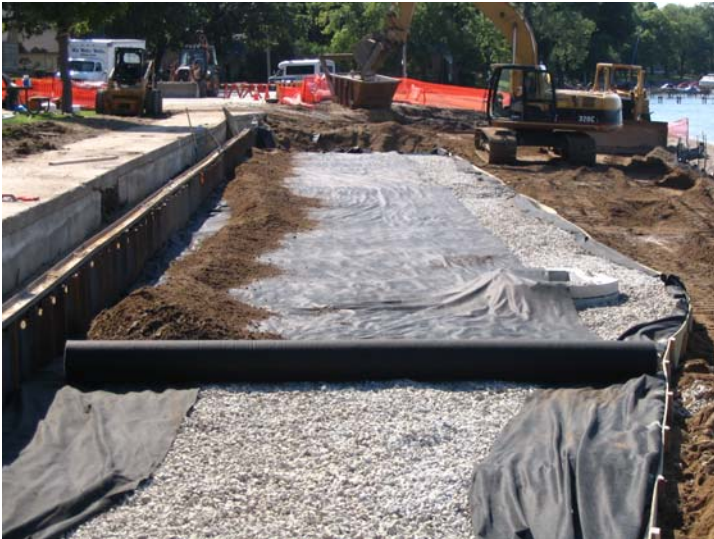
Infiltration Trench (Previous Project)
