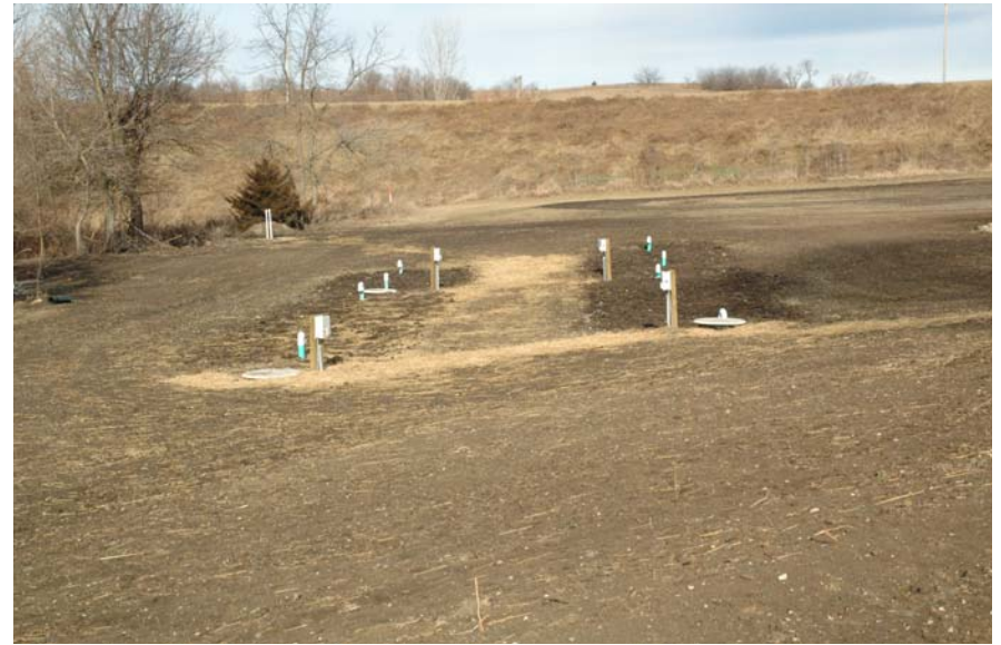
Completed earthwork and new seeding.
