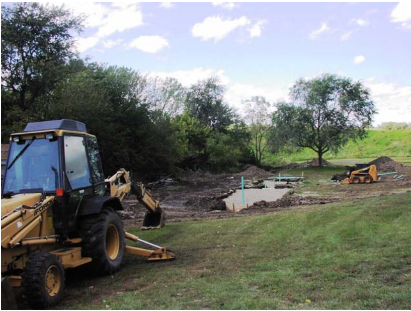
Installation of the sand filters and dosing tank.
