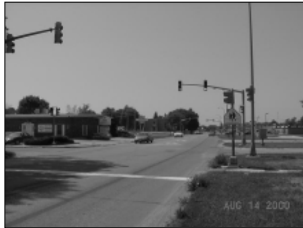
Figure 14 Missing Crosswalks at Intersection 26
