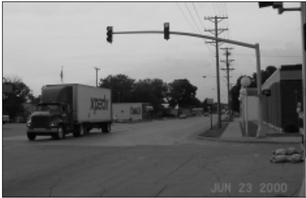
Figure 1 South Leg of Intersection 01
