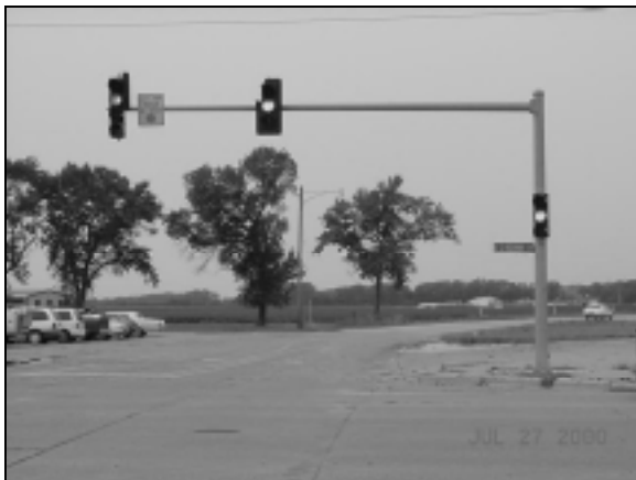
Figure 9 Damaged Backplates at Intersection 14
