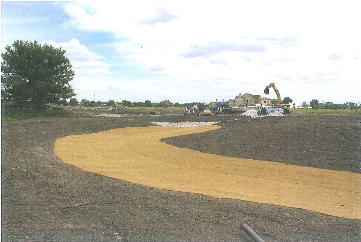
West Bioswale During Construction
