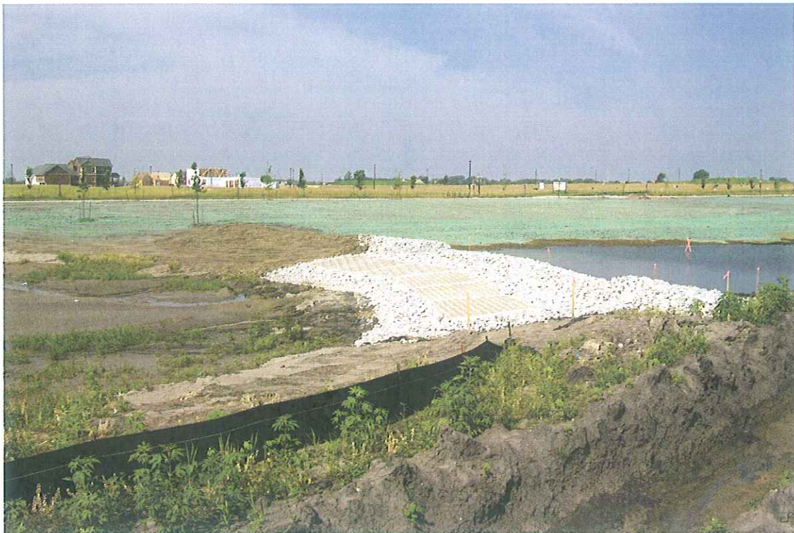
Forebay weir with maintenance crossing
