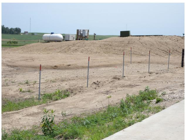
This media filter system recirculates the community's wastewater until treatment is achieved and then is treated again with Ultra-Violet disinfection and discharge into the Middle Raccoon River.
