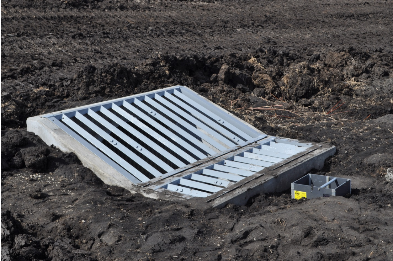
Concrete Riser with water control structure
