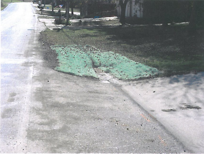
Photo 7 A completed bio-swale without vegetation planted yet but fiber mulch.
