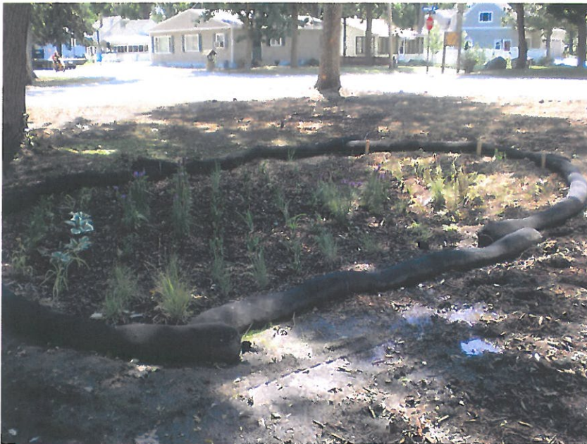
Photo 8 Completed Bio-Cell with protective fiber log until establishment.
