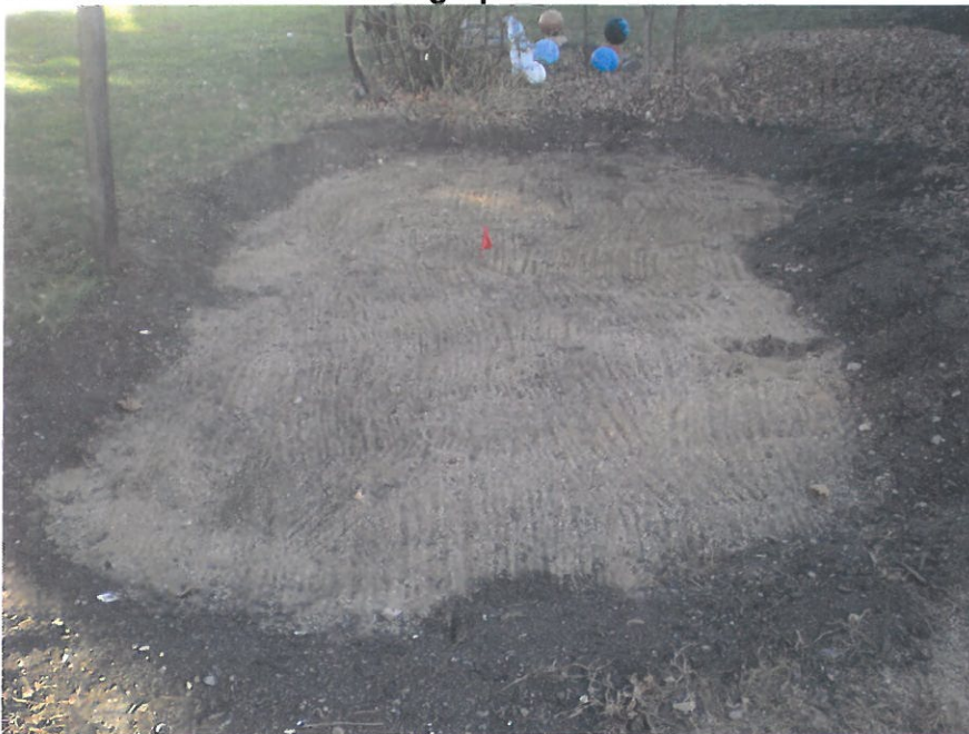
Photo 4 Rain Garden as constructed with no vegetation planted yet in Spirit Lake
