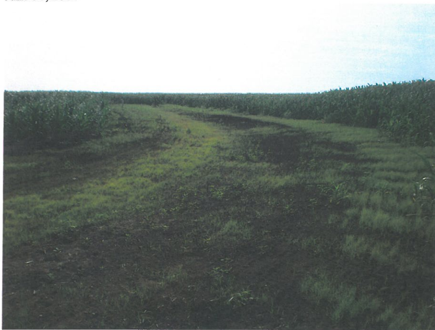
Photo 15 Same gully as Photo 14 after shaping and seeding of Grassed Waterway
