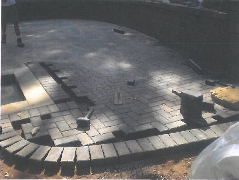
Photo 5 Pavers being placed and constructed. The underlayment is already in place.
