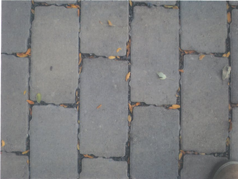
Photo 6 Another Paver Project complete with proper spacing and filler
