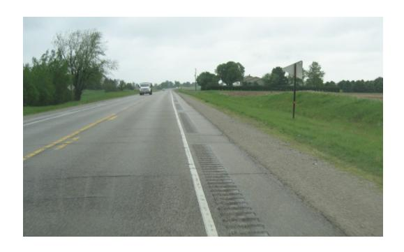
Figure A.27. US 151 pavement conditions with paved shoulder rumble strips
