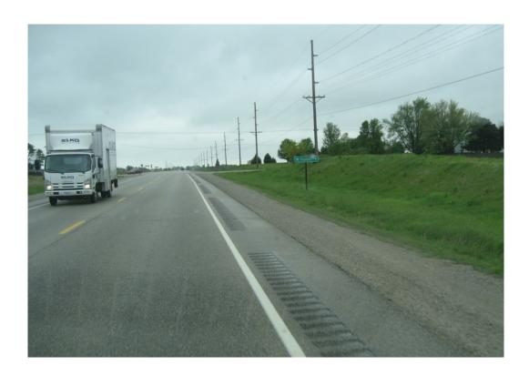
Figure A.28. US 151 pavement conditions with paved shoulder rumble strips
