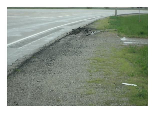
Figure A.7. Shoulder edge deterioration near Norway Road intersection
