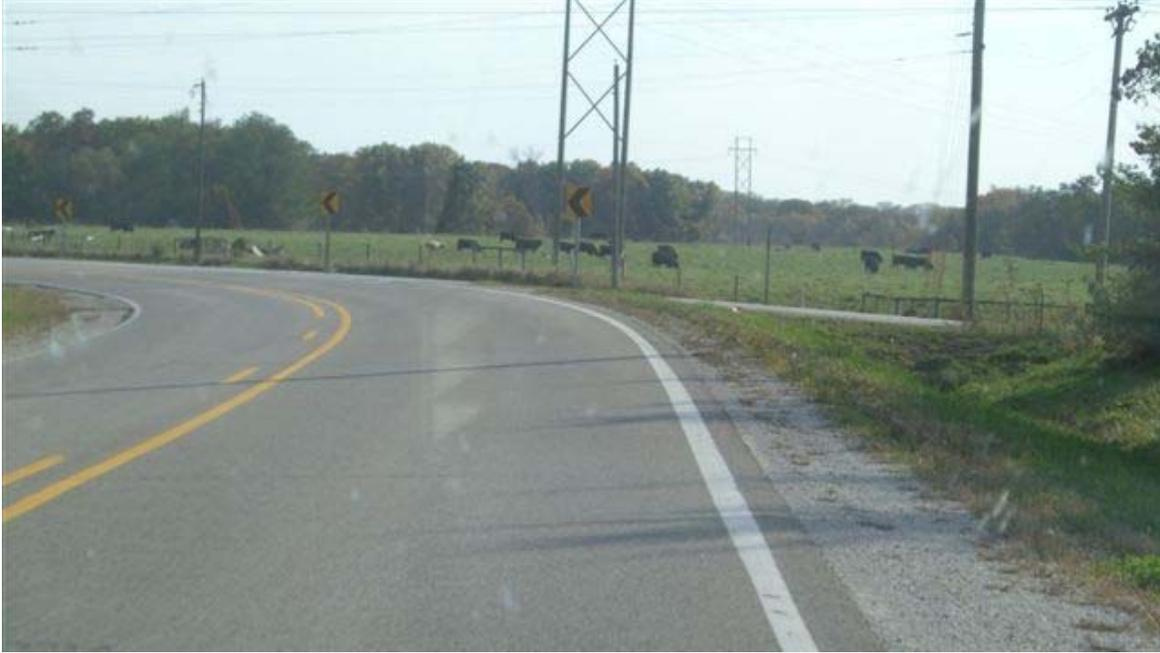
**Figure A.5. County Road X-23, chevron installation along horizontal curve**
