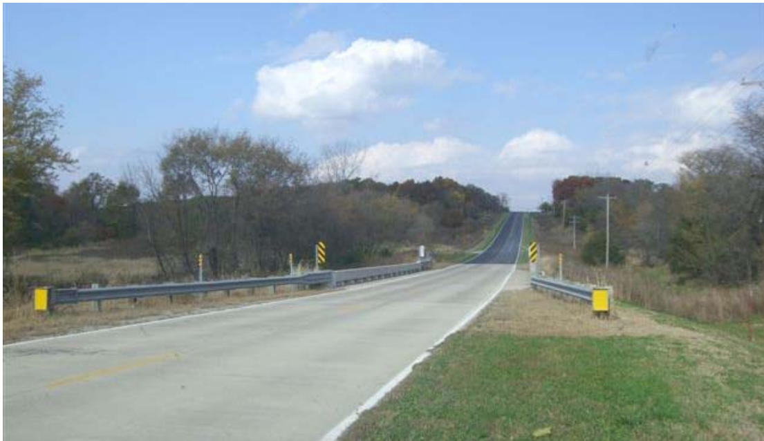
Figure A.6. Guardrail and delineation at newer bridge
