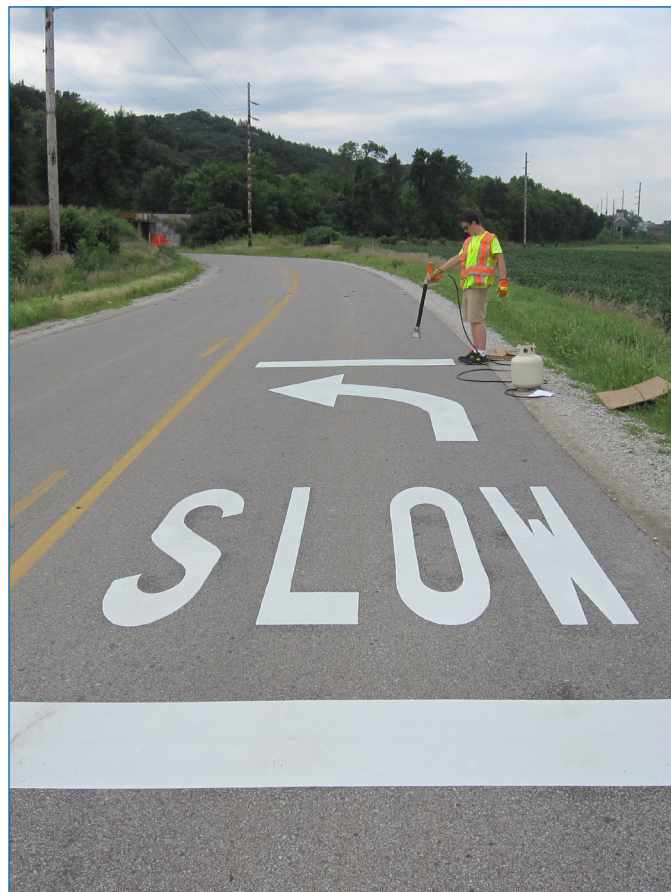
Use of a blow torch to attach thermoplastic pavement markings on CR L20
