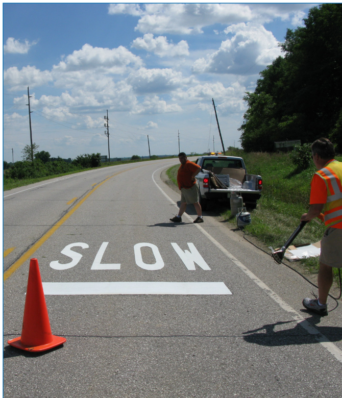
Installation of supplementary on-pavement markings on DMC 99
