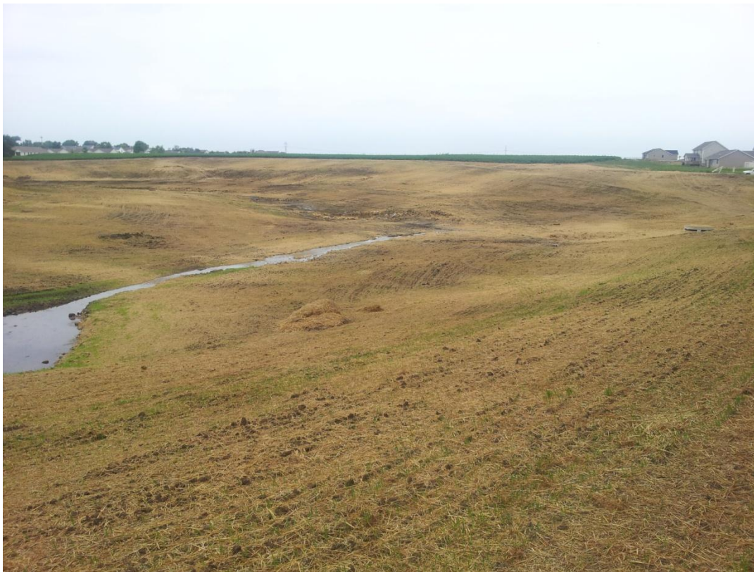
Temporary seeded and mulched finished basin
