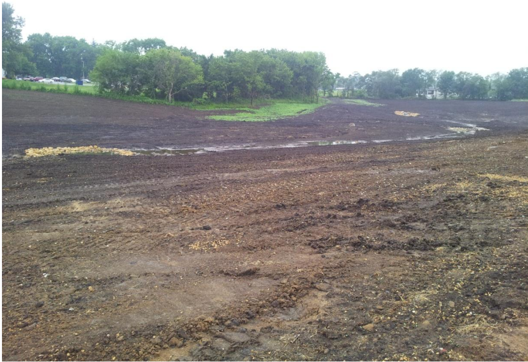
Graded basin with pools and riffles
