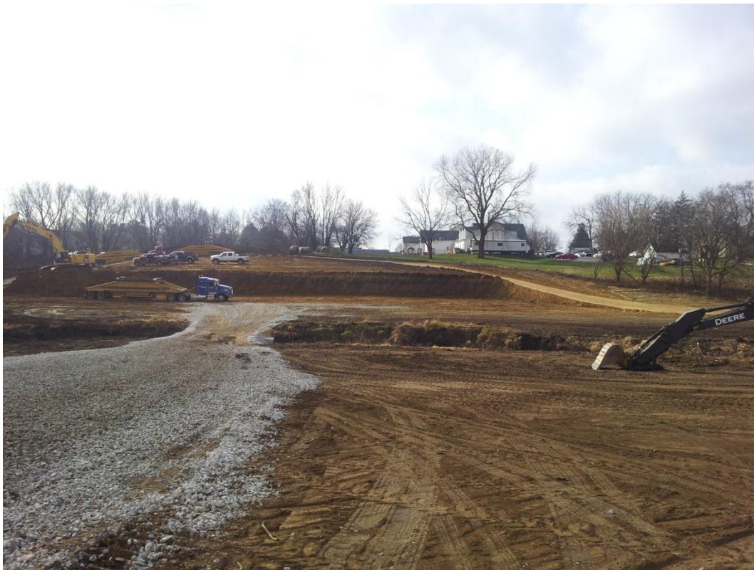
Excavation of the south side of the basin
