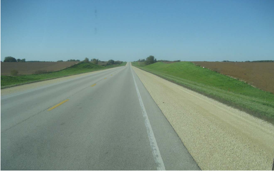
Figure D.31. US 52—Winneshiek County partial paved shoulder
