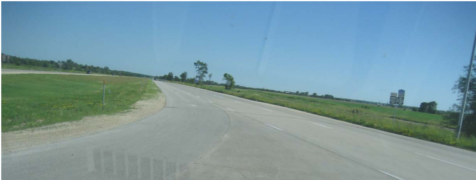
Figure B.11. Left-turn acceleration lane on southbound US 218
