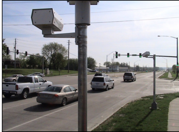
Figure 3.6. RLR camera system monitoring eastbound traffic at 156th St. & Hickman Rd.
