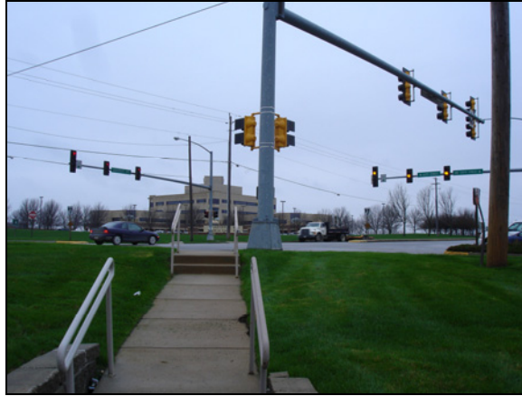
Figure 3.24. Westbound traffic for 60th St. & University Ave.
