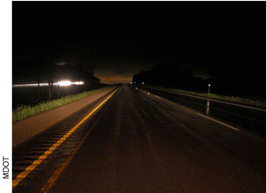
Figure 1.2. Nighttime view of edgeline rumble strip (image source: http://www.tfhrc.gov/pubrds/06jul/images/morena14.jpg )
