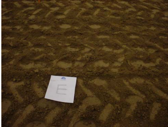
Figure 37. Surface condition after compaction for Test Strip E
