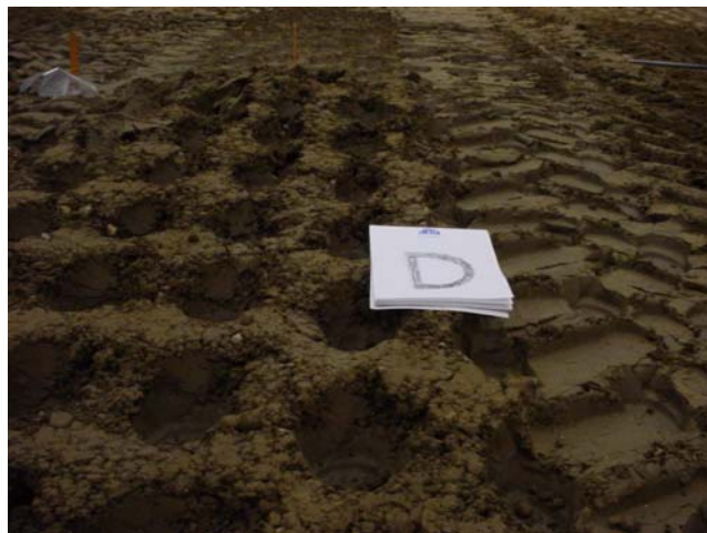
Figure 36. Surface condition after compaction for Test Strip D
