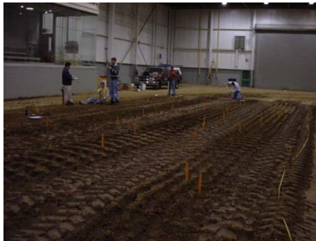
Figure 33. Test strips A through D after compaction
