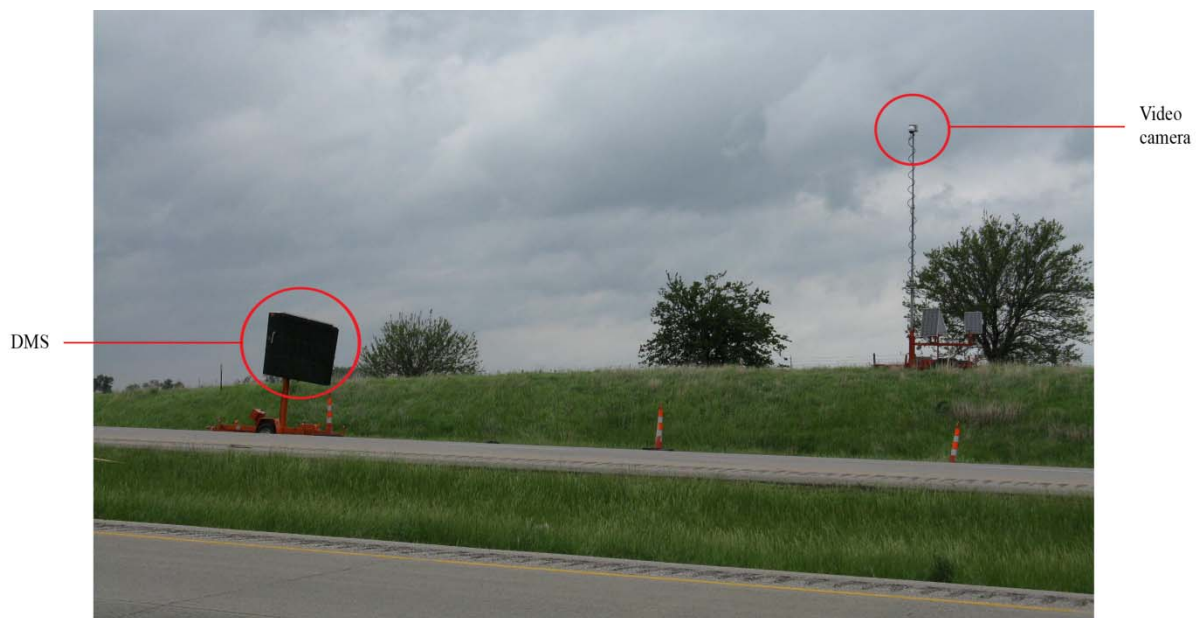
Figure 4. Typical installation (may include the DMS, left, and sometimes a solar-powered video camera, right) (photo courtesy of Iowa DOT)
