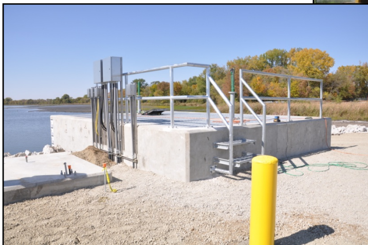
New 20,000 gallon per minute pump station
