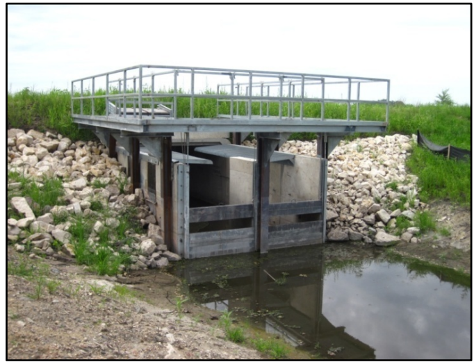
The new outlet and water control structure at Pickerel Lake (above). Fish barriers on the outlet structure at Pickerel Lake (left). These overhanging fingers allow debris to flow over the barriers but keep carp from jumping up into the lake from downstream. Note the barriers on the stop logs can move up and down with the elevation of the logs.
