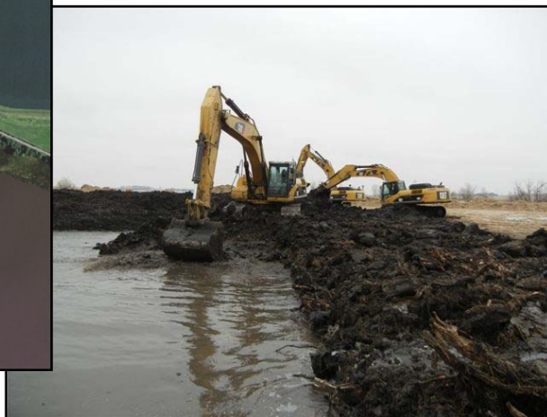
Serpentine channel excavation at the inlet of Little Storm Lake
