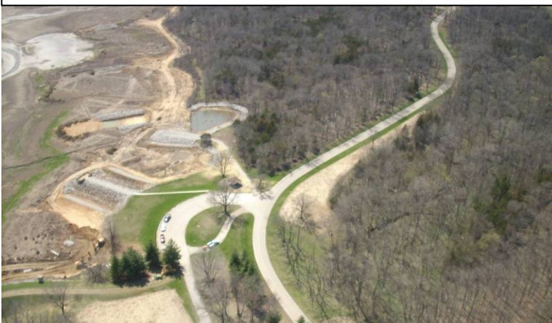
Lake Wapello during 2009 drawdown for in-lake habitat work, shoreline stabilization and outlet valve replacement
