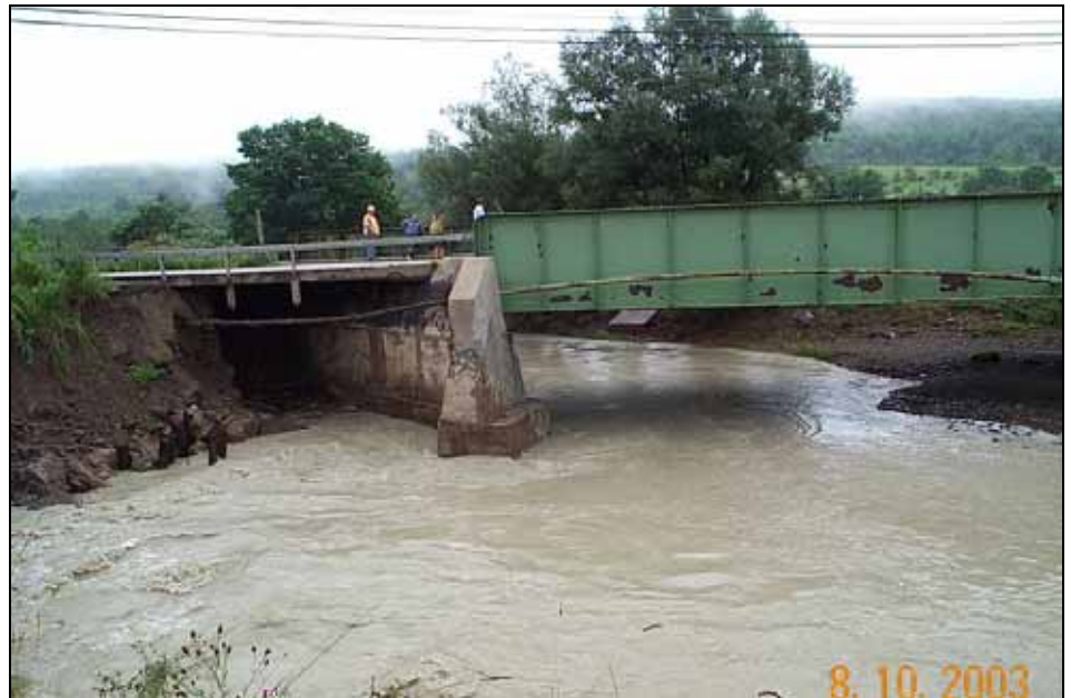
Waterway scour threatens bridge abutment and embankment.
