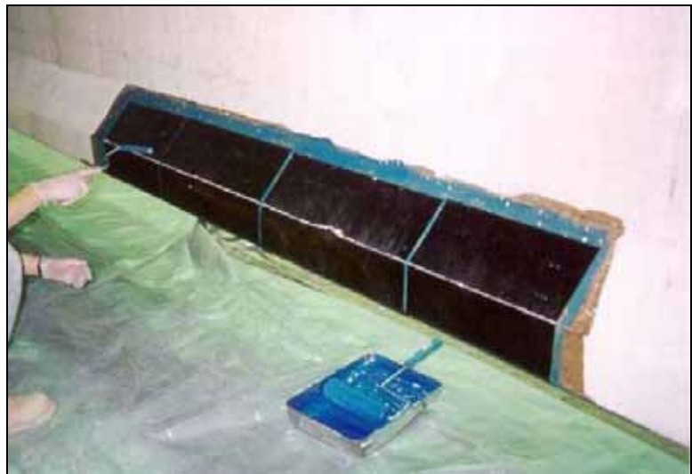
Installation of transverse CFRP jacket on Beam
