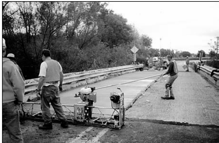
PCC Placement on the Independence Bridge
