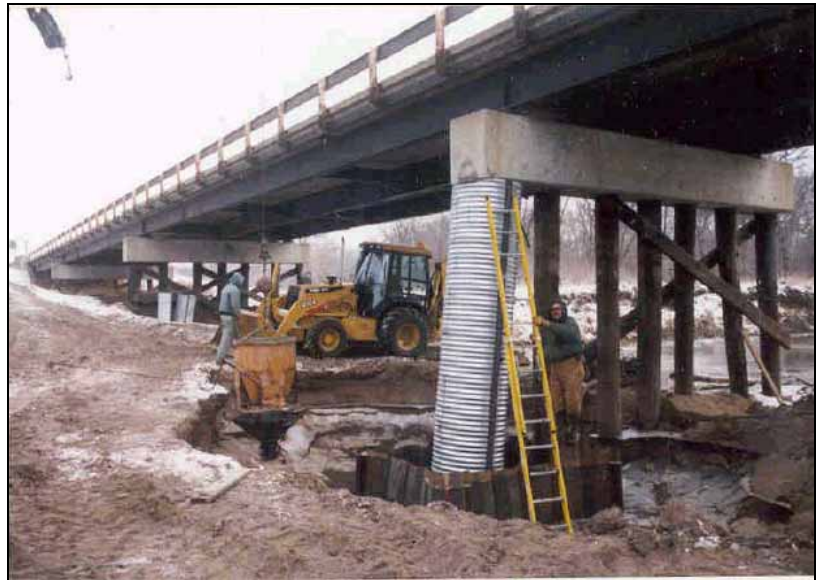
Jacking of Deteriorated Timber Piles
