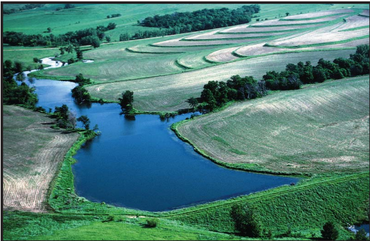
A watershed dam and upland terraces in a small watershed project in western Iowa. Photo: Iowa NRCS.
