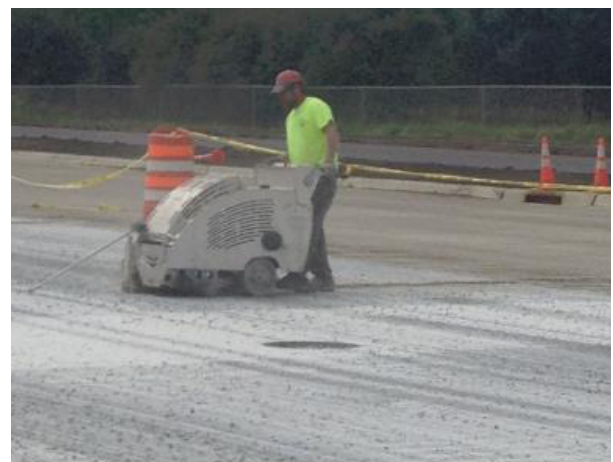
Typical early entry saw-cutting process
