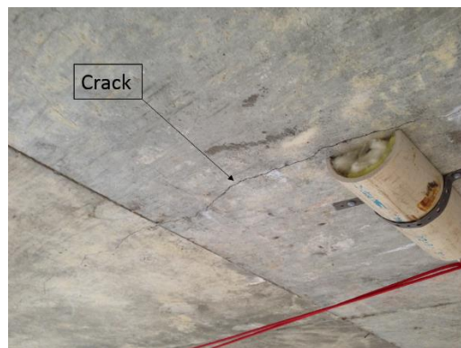
Figure 45. Relative positions of crack and strain gauge in the fifth bay
