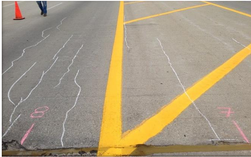
Figure 5. Longitudinal cracks at the center of the south end
