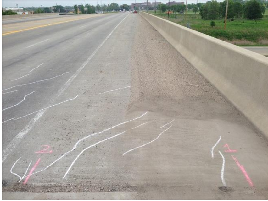
Figure 6. Diagonal cracks at the corner of the deck
