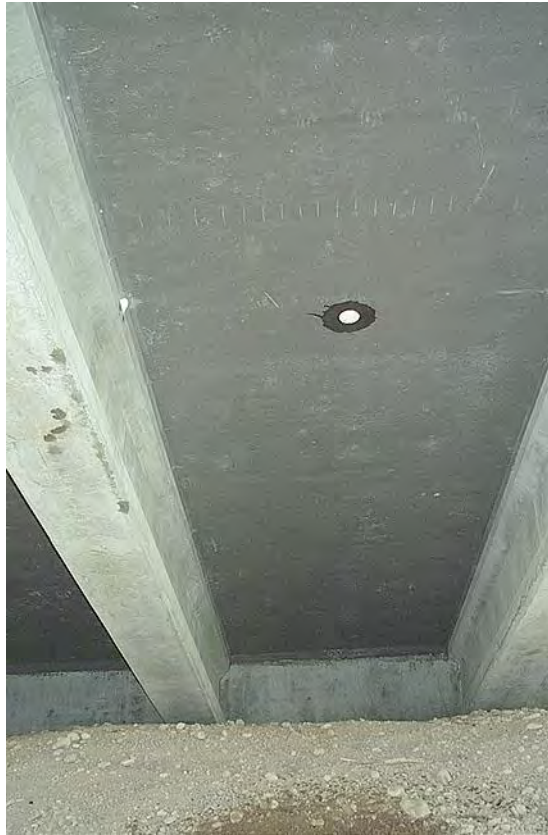
Figure A2.113. Photograph from beneath bridge deck after coring operation, hole from core S-1 is clearly visible, light coming through hole from core S-2 is partly obscured by the pre-stressed beam.
