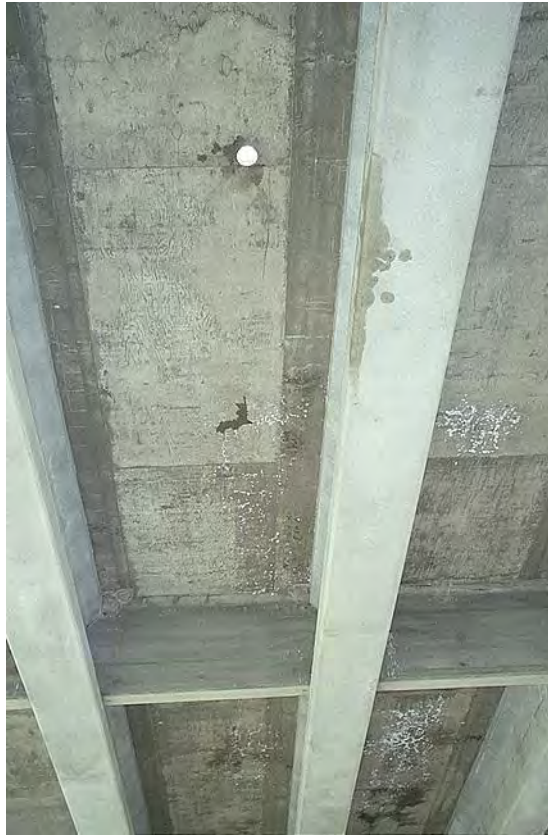
Figure A2.97. Photograph from beneath bridge deck after coring operation. Hole from core T-2 is visible. Dampness permeating through cracks visible beneath the area of core T-1. White efflorescence common in areas directly below regions covered with cold patch material.
