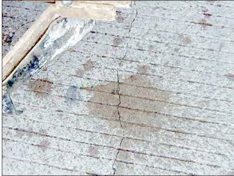
Figure A2.19. Photograph of crack in bridge deck.
