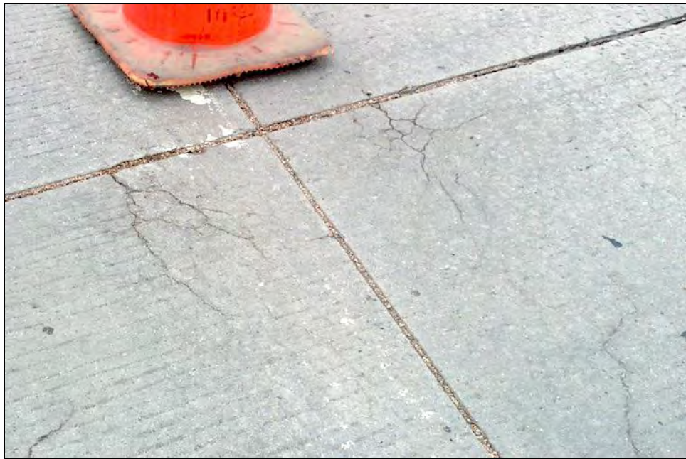
Figure A2.1. Photograph of cracks in pavement.
