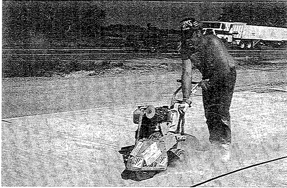
Figure 1 Sawing Beveled Edge on Longitudinal Joint
