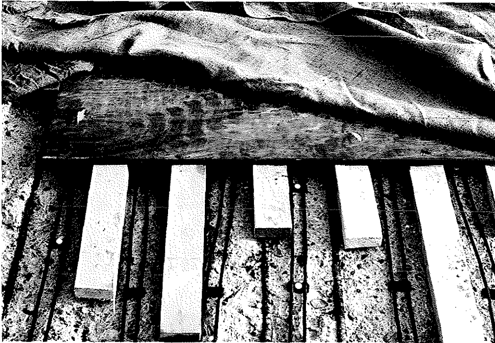
Figure 10 - Bridging over large repair area
