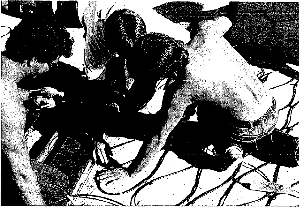
Figure 8 - Hand woven ends at raised plates
