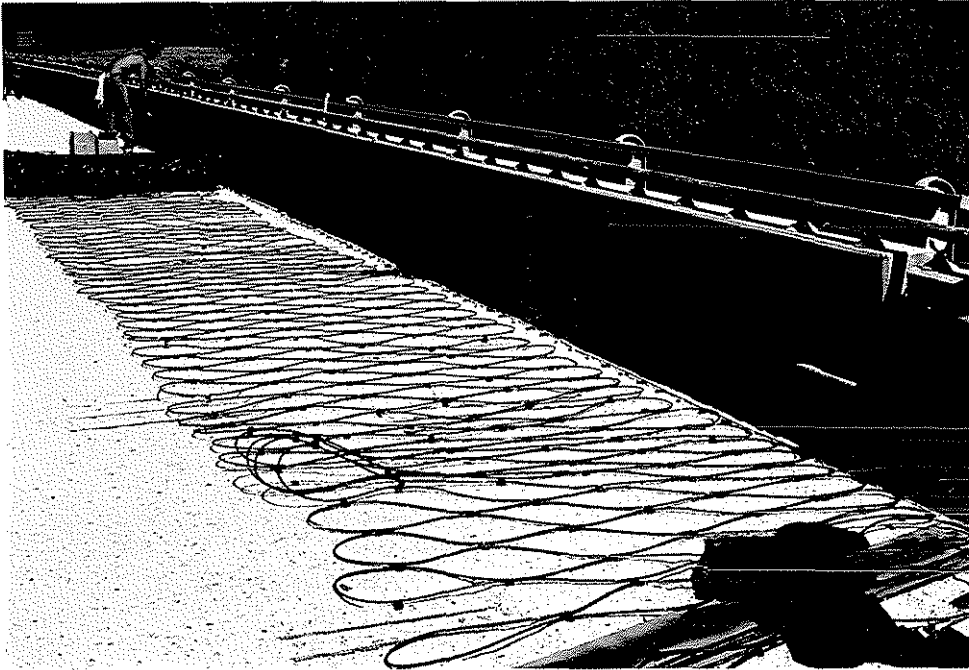
Figure 4 - Rolling out first anode mat
