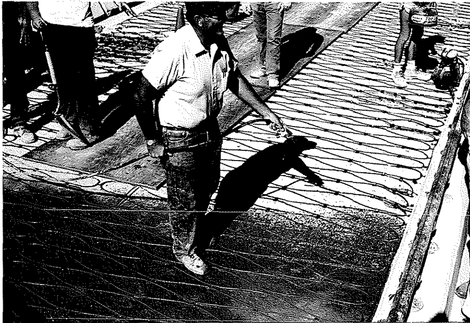
Figure 11 - Grout spraying
