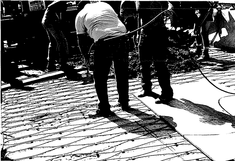
Figure 12 - Puddling in front of paver
