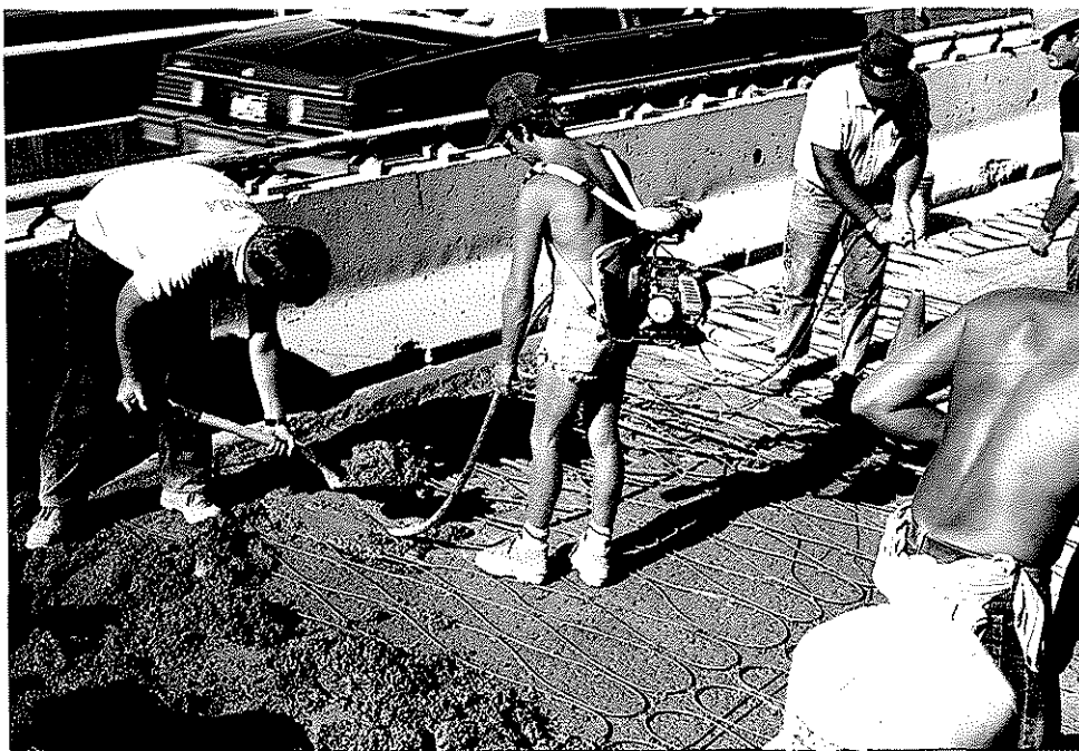
Figure 13 - Filling and vibrating small repair area
