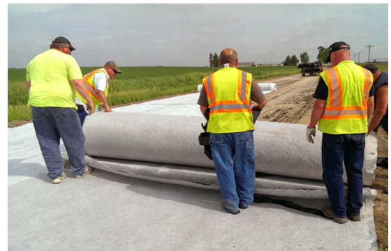
A geocomposite drainage layer was placed at the aggregate-subgrade interface in Section 18
