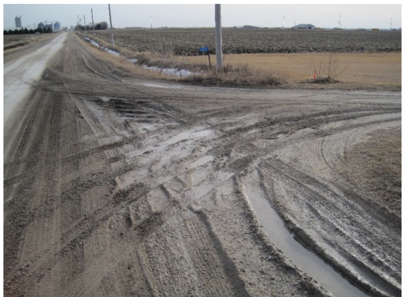
Post-thawing conditions of selected road before stabilization
