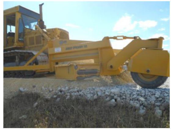
An aggregate spreader was used to place the macadam base and surface course materials
