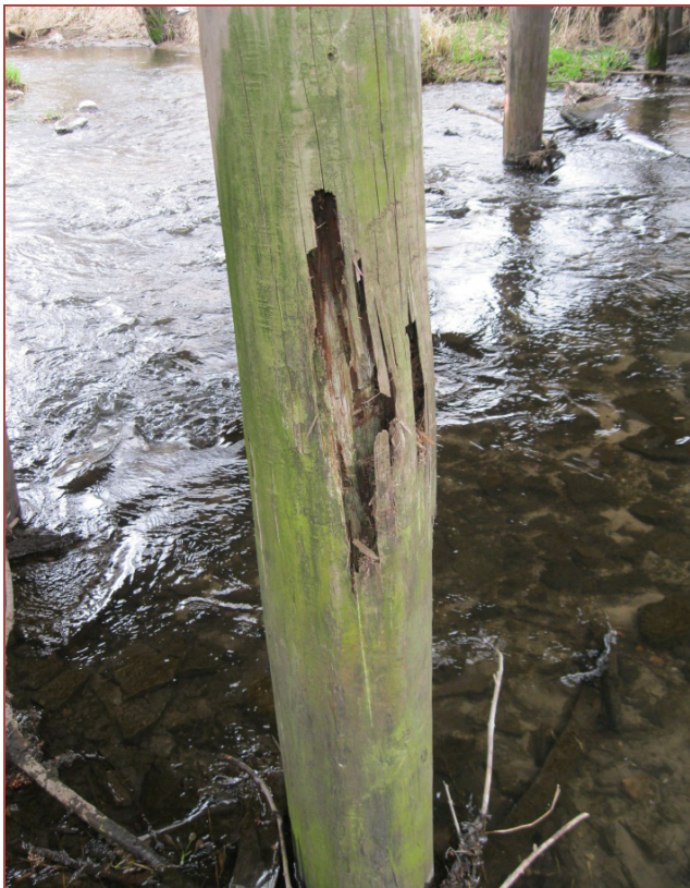
Sample damage and decay at demonstration project
