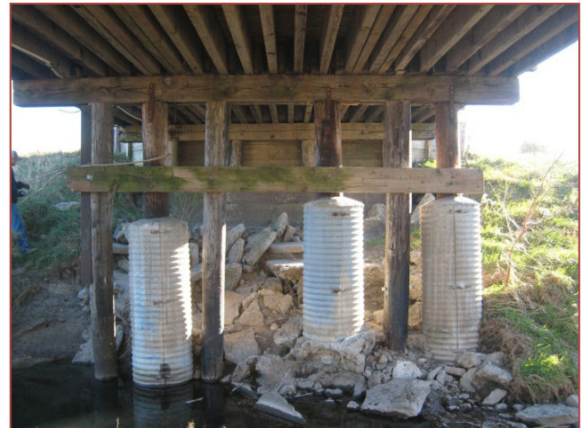
One variation of casts created from corrugated metal pipe (CMP) and concrete infill
