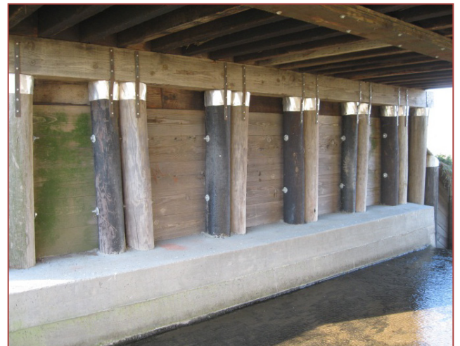
One variation of new concrete sills and pile caps
